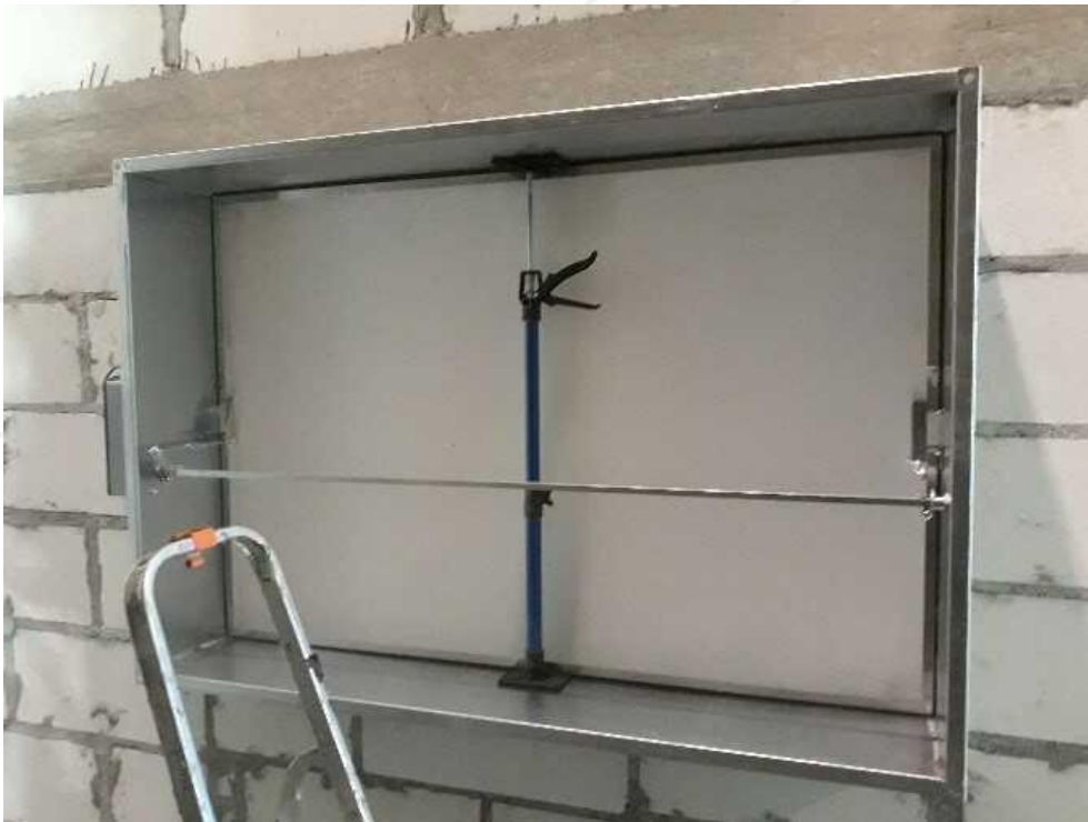
Figure 1. Correct preparation of the damper for the installation (using spreader securing the housing)
