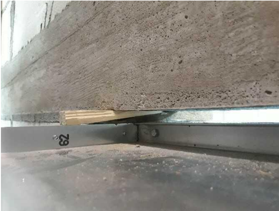
Figure 2. Correct preparation of the damper for the installation (using mounting wedge)
